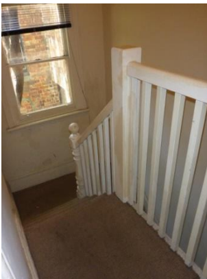
Picture 9 – View down the staircase in the dwelling at 196 Oxford Street
