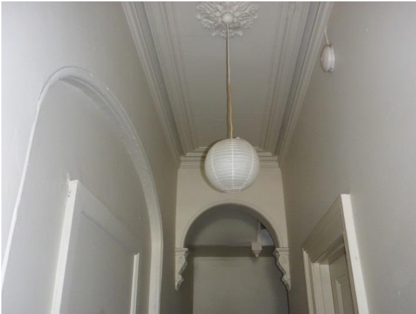
Picture 7 – View of the central hallway of the dwelling at 196 Oxford Street
