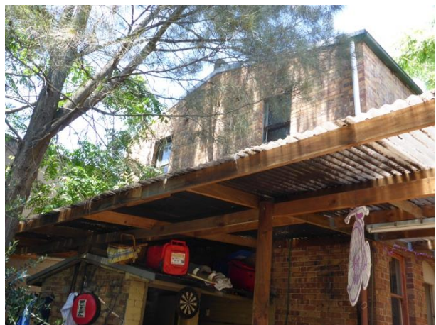
Picture 6 – View south east at the rear façade of the dwellings at 198-200 Oxford Street
