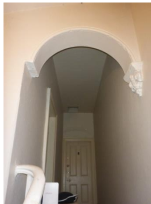
Picture 10 – View up the central hallway on the first floor in the dwelling at 196 Oxford Street
