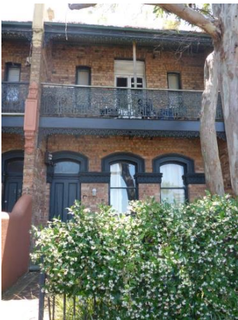
Picture 3 – View north towards the primary (southern) facade of 196 Oxford Street
