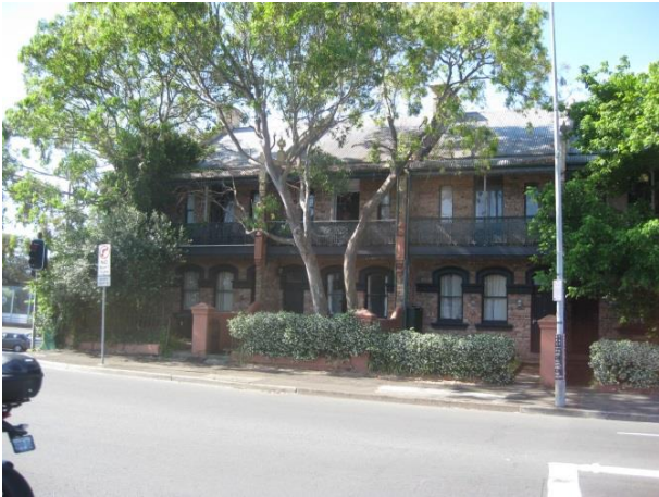
Picture 1 – View north towards the primary (southern) facades of the subject dwellings
