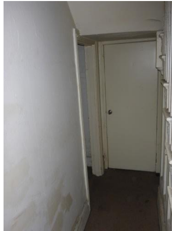
Picture 8 – View of the central hallway of the dwelling at 196 Oxford Street
